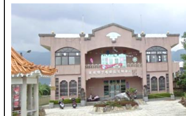
Made by Yilan County Fire Dep.
